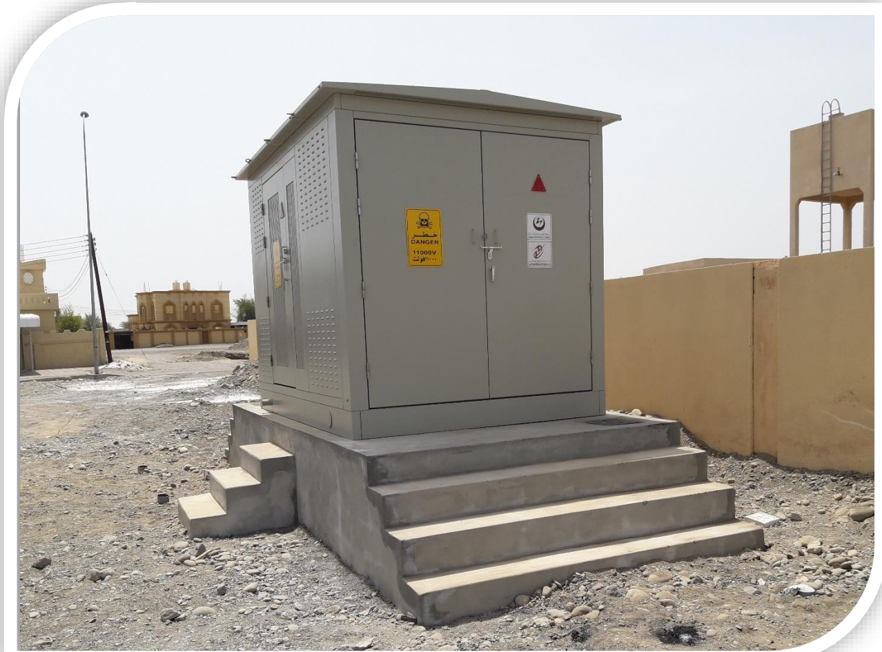
Installation of Package Substation
