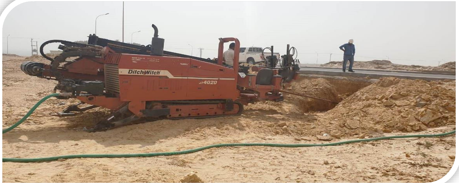
Preparation at sites for Horizontal Directional Drilling
