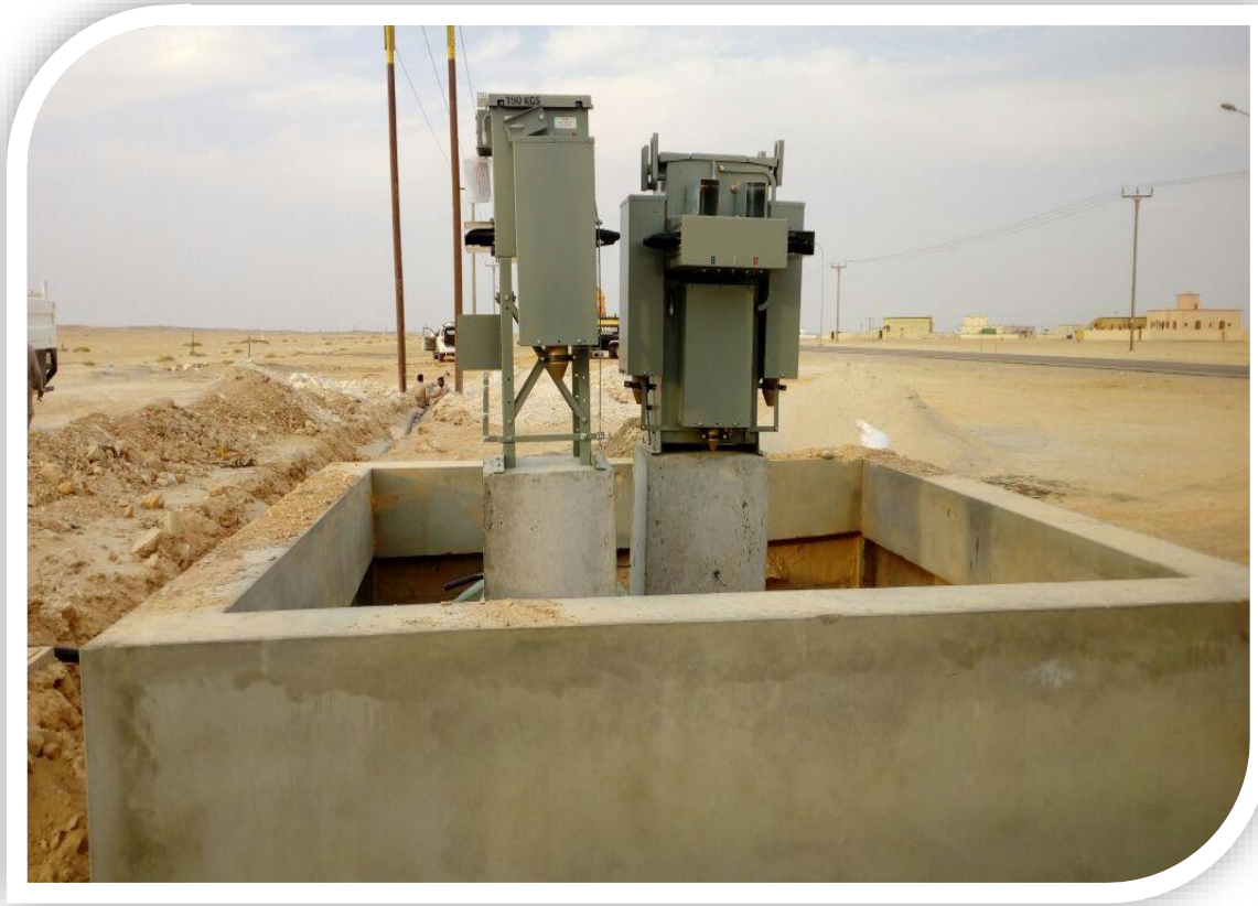
Construction of Fiberglass Type 11kV Substation
