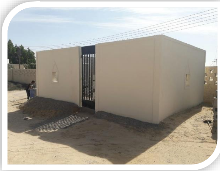
Construction of wall type 11kV Substation
