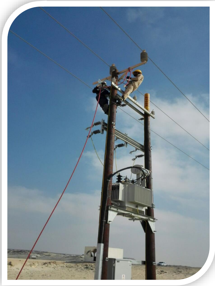
Work in progress on LV and 11kV Overhead Lines
