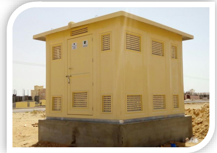
Construction of Fiberglass Type 11kV Substation
